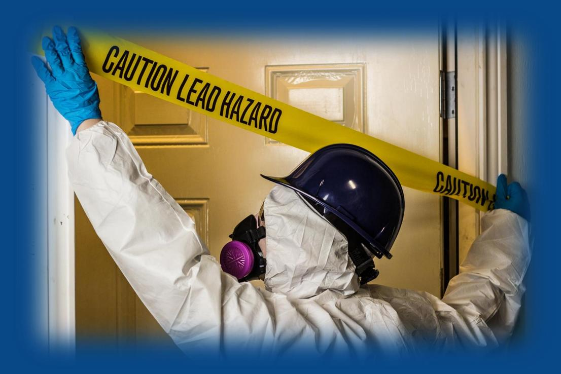
In certain cases, interim controls are unlikely to be effective, especially if the building has substantial structural defects or if interior or exterior walls, or major components, are seriously deteriorated or subject to excessive moisture. In these situations, abatement is more appropriate in addressing leadbased paint hazards.
