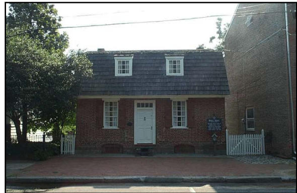
Figure 18: The Revell House
